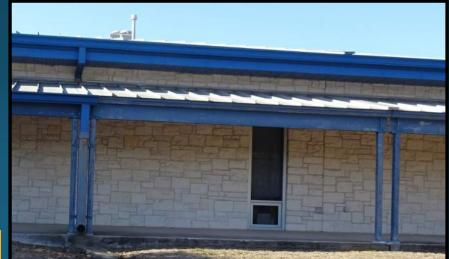
Downspouts, Gutter Expansion Joints
